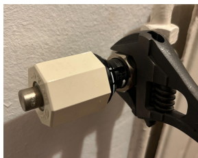
Skruva loss termostaten
